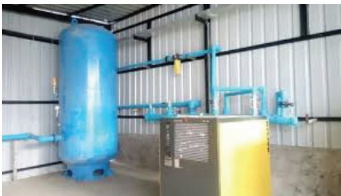
Figure 32: HDPE Aluminium Pipe line
