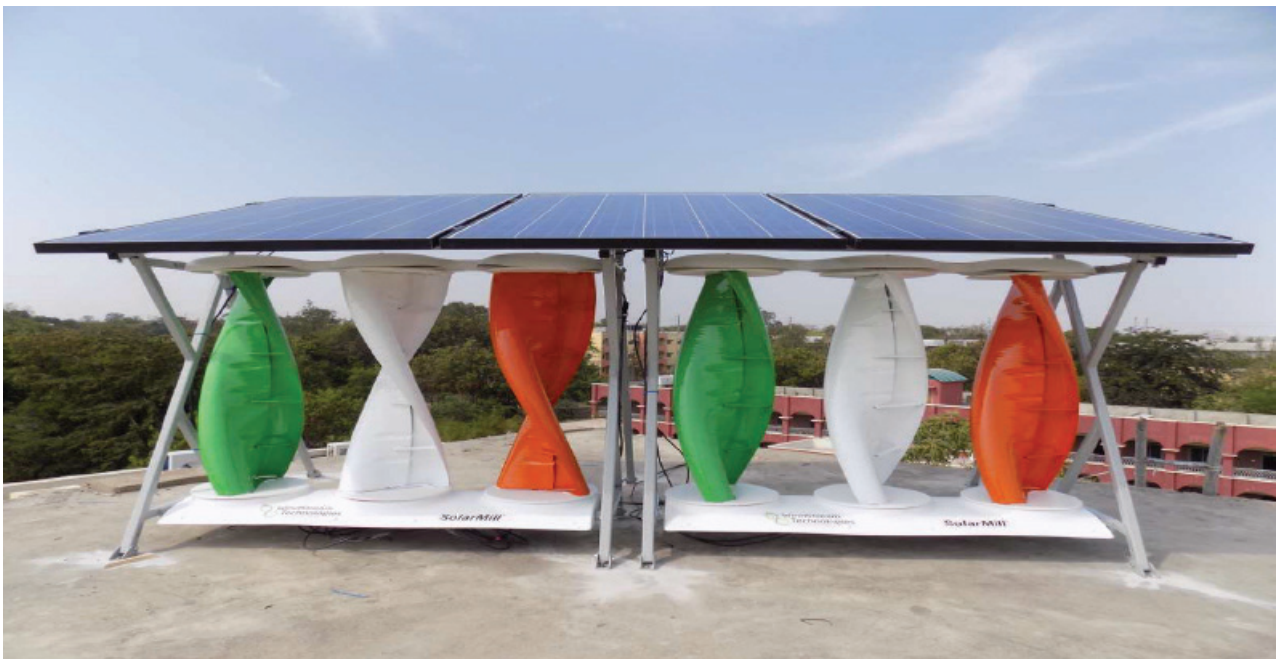
Figure 43: Solar wind hybrid system
