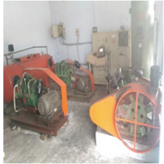
Figure 30: Reciprocating Compressor
